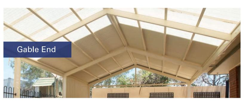
The Fielders Centenary Gable End range is engineered for strength. Available in both 108mm and 158mm portals which allow for gable widths beyond 10 metres. The gable unit can be attached to an existing structure or installed as a freestanding unit. Centenary's gables are available in 15, 20, 25 or 30 degree roof pitches, the greatest variety of pre-engineered gables on the market today.
